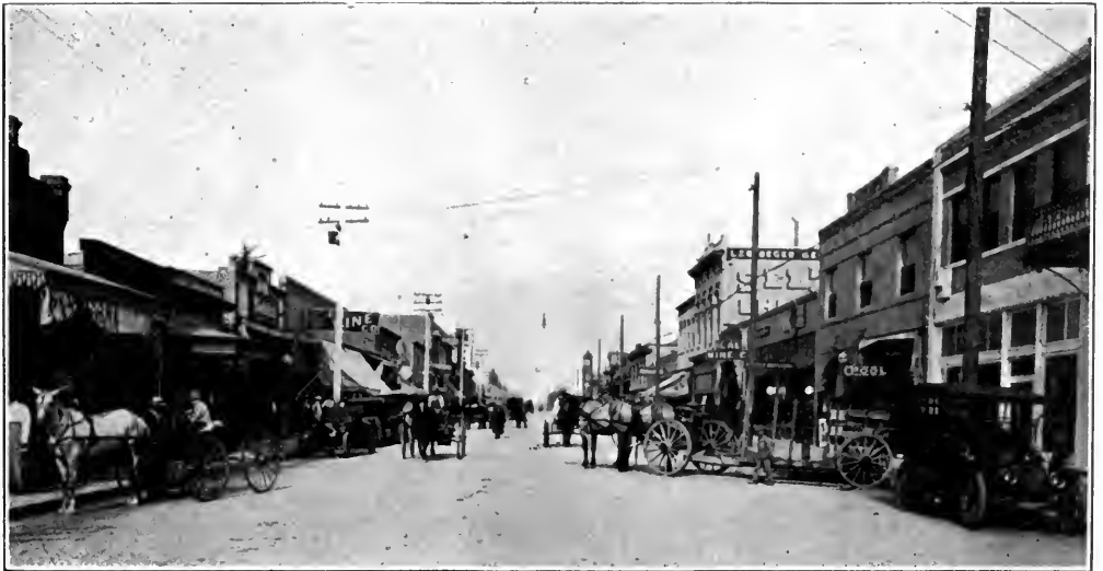
Center Street, Anaheim, Looking East.
